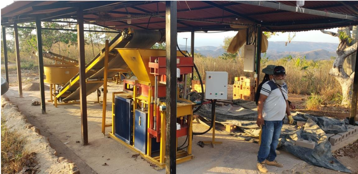
Figure 3: Productive unit and hydraulic press to produce Compressed Earth Blocks in Tierra Grata. Photo: Daniela Sanjinés
